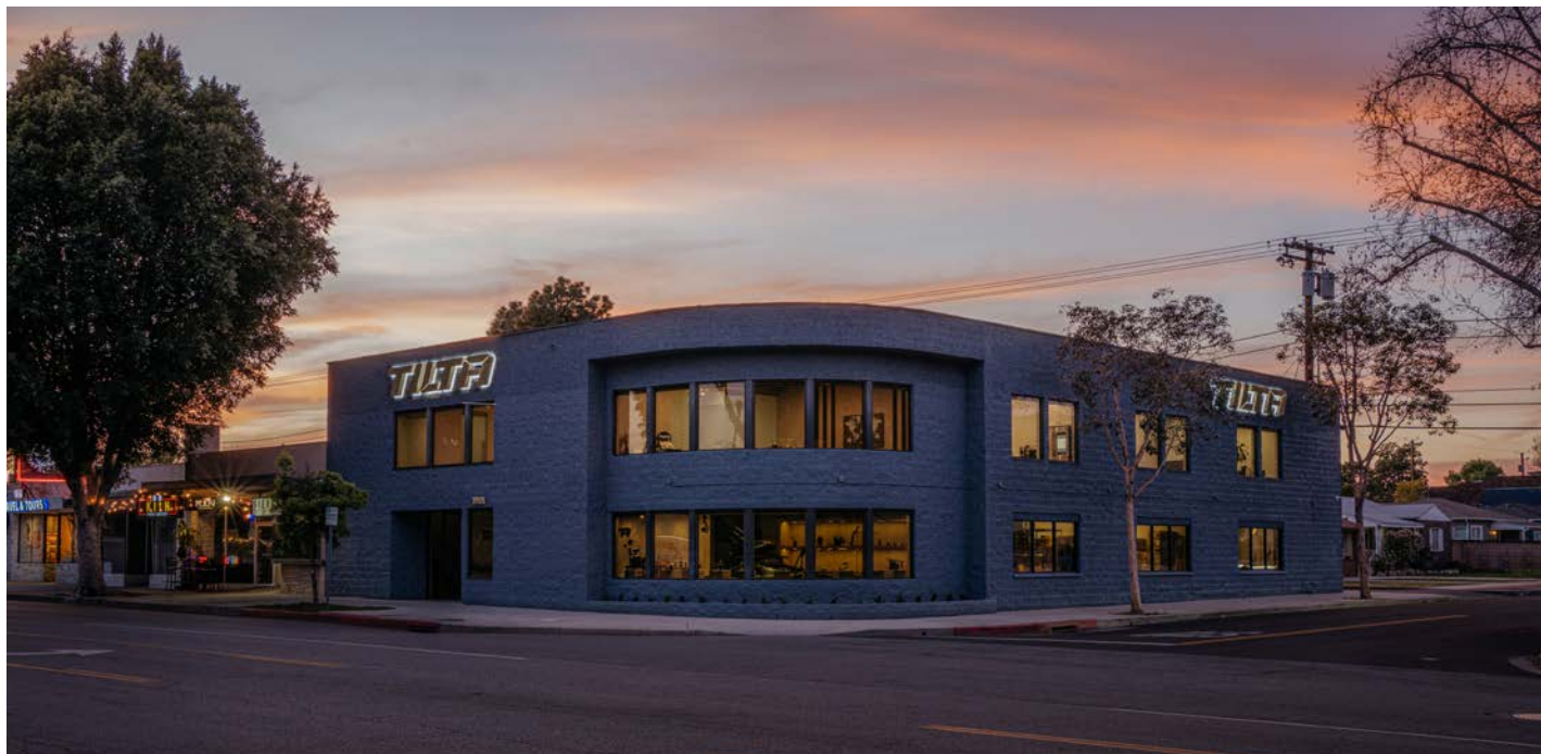
Above: Tilta Burbank at magic hour. Below: Showroom and Lobby.
